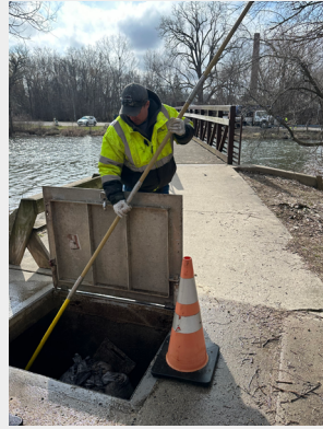
Pictured: Wastewater Operators Phil Z. and Mark B. clean out the inverted siphons that carry wastewater underneath the Yahara River.
