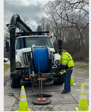
Pictured: Wastewater Operators Phil Z. and Mark B. clean out the inverted siphons that carry wastewater underneath the Yahara River.
