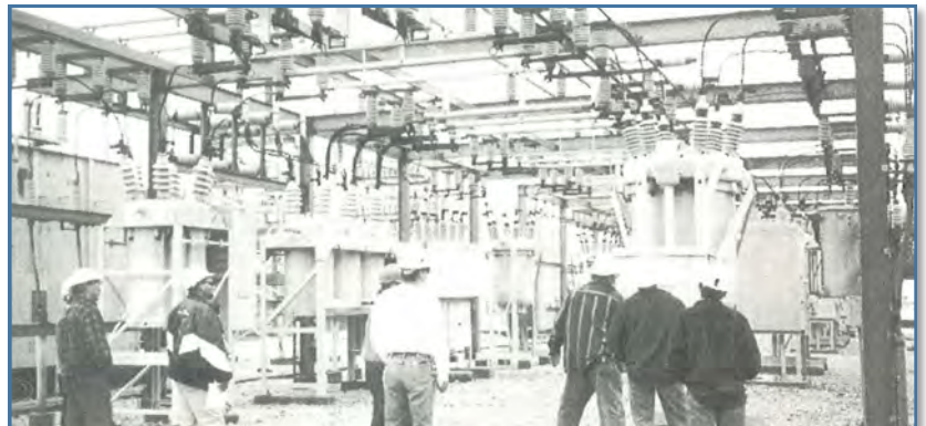
Substation Workshop attendees walk through a WEPCO facility in 1998.
