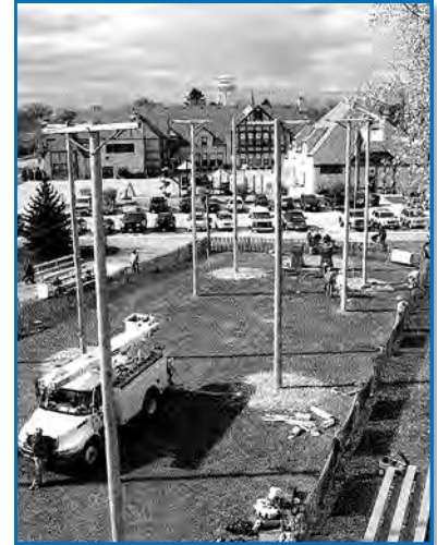
First Lineman’s Rodeo held in Menasha at Jackman Park.
