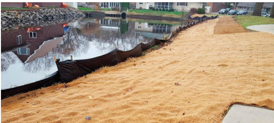
The City of Monona completed a shoreline restoration project.
