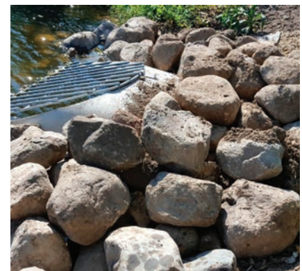
Monona also upgraded a stormwater outfall.
