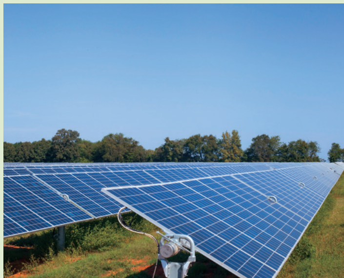
The Point Beach Solar Energy Center will use solar photovoltaic panels similar to the ones pictured from the River Bend solar site in Florence, Alabama to convert sunlight into electricity.
